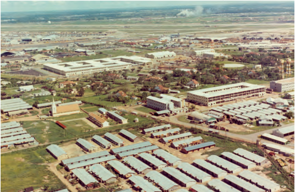
The MACV headquarters complex at Tan Son Nhut (the airfield is in the background) was completed by RMK-BRJ in the summer of 1967.
